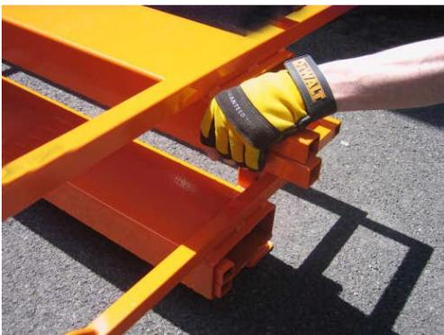
Turn the wing bolts anticlockwise until the threaded bolts are clear & the pillars can drop fully to the base of the sockets
